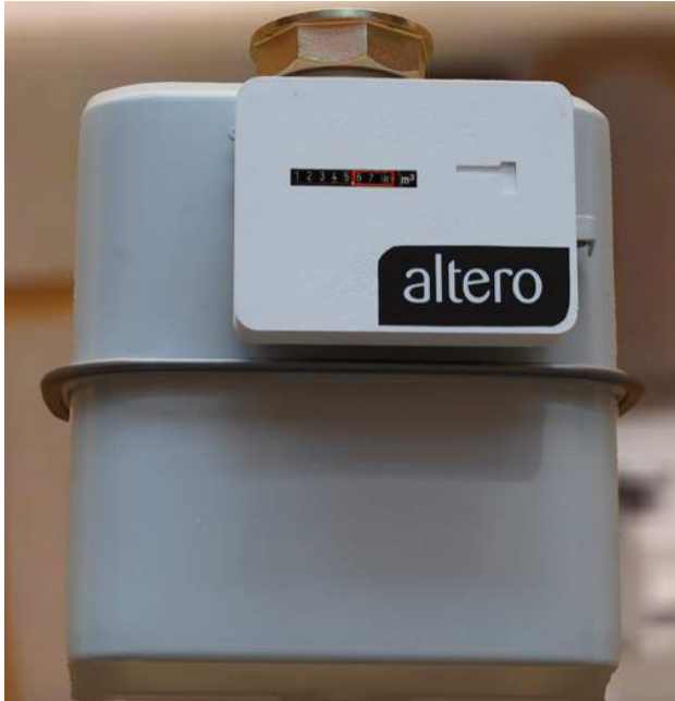
The MeterCam installed on a gas meter.
